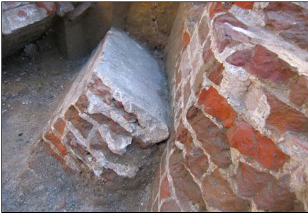
Figure 111: Section of parapet with finished surface.
