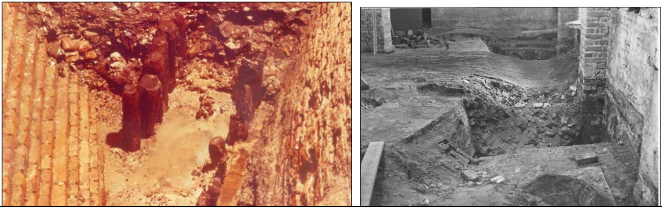
Figure 122: Excavations of the Half Moon in basement of the Exchange; wood planking and pales at base of the foundation.
