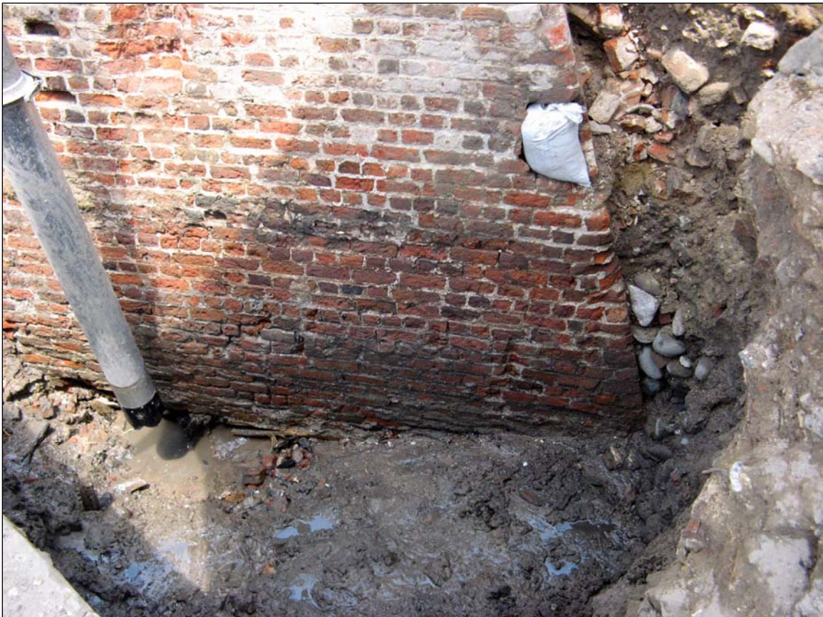
Figure 47: Excavations to the base of the brick redan, below water table, with aid of the vacuum truck.
