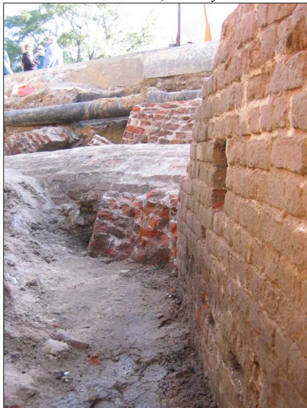
Figure 107: North face of redan, showing sections that are vertical (foreground) and battered (background). Demolished parapet sections are visible in front of the battered portion.
