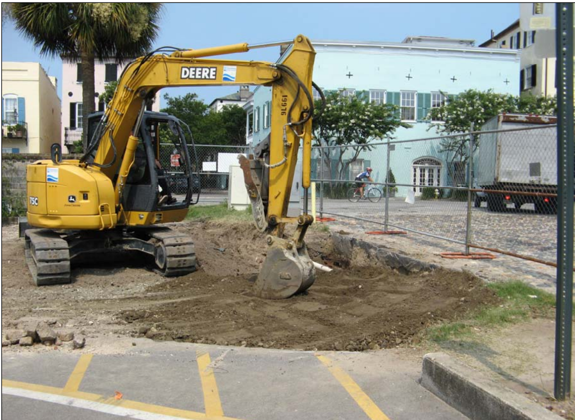
Figure 48: Backfilling of 2009 excavations by Charleston Water Systems.
