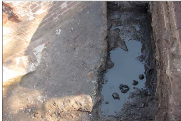
Figure 114: Row of pilings parallel to face of redan.
